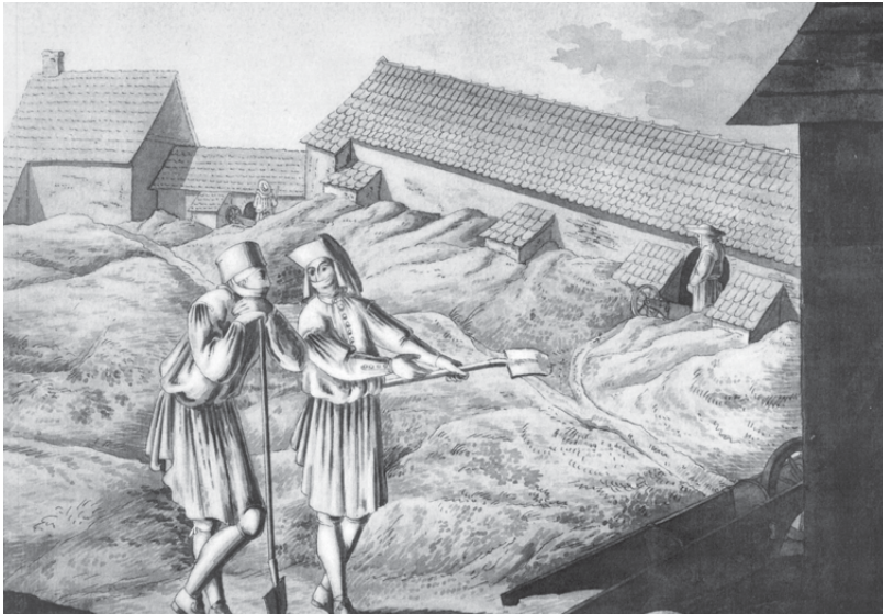
Figure 7. The large amount of accumulated toxic waste (mostly arsenic oxide) that has collected in the smoke chambers is scooped out by workers wearing mouth masks.
